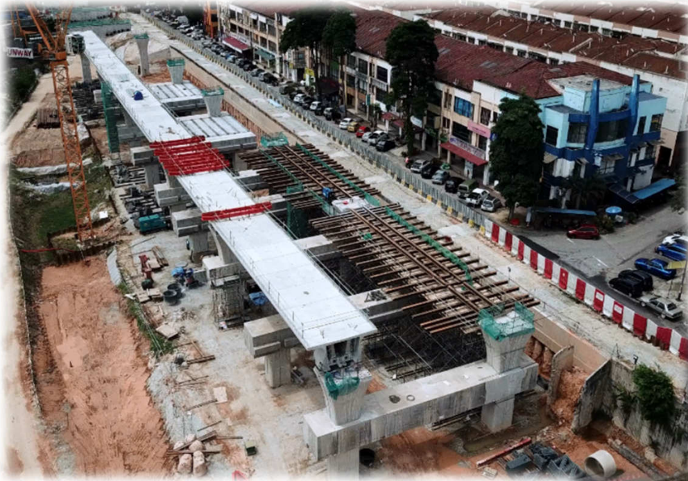
Damansara Damai Station
