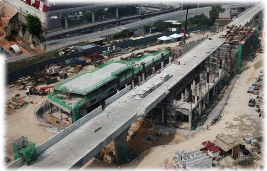
Damansara East Station
